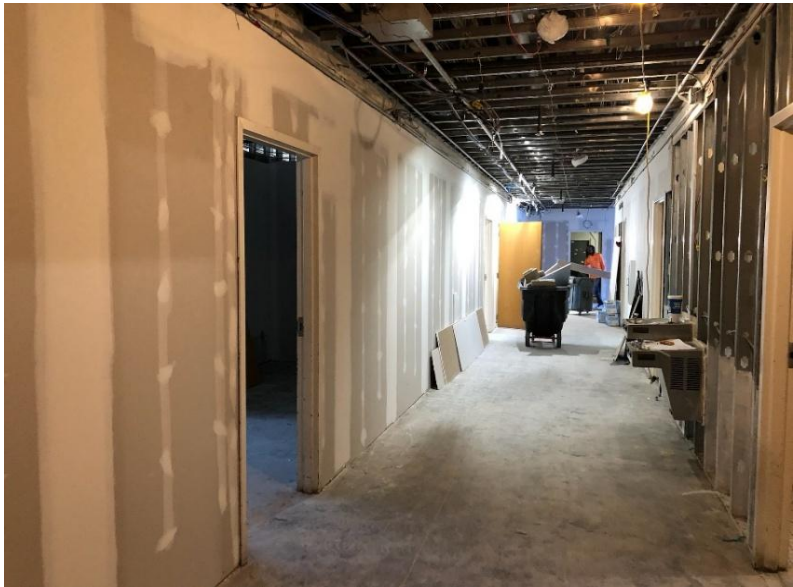
Parkview First Floor Renovations
