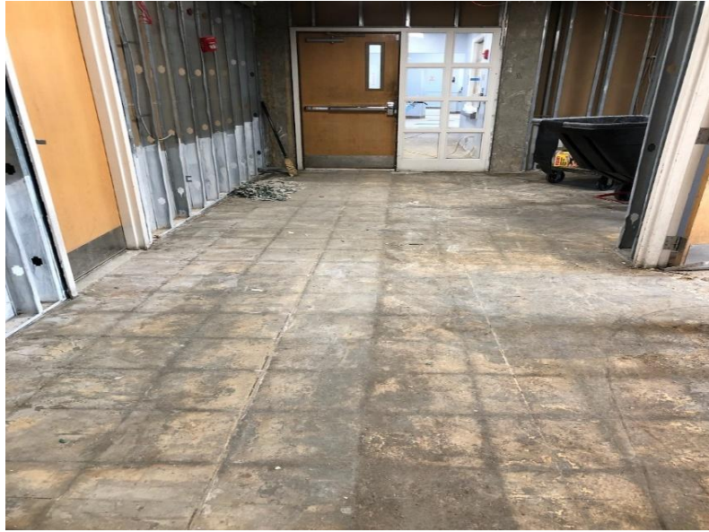
Parkview First Floor Renovations
