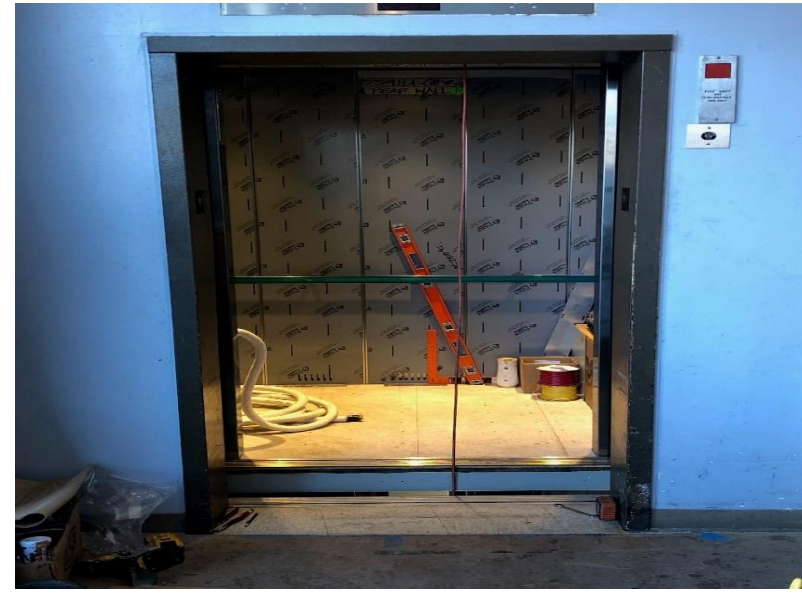
Parkview Elevator Replacment
