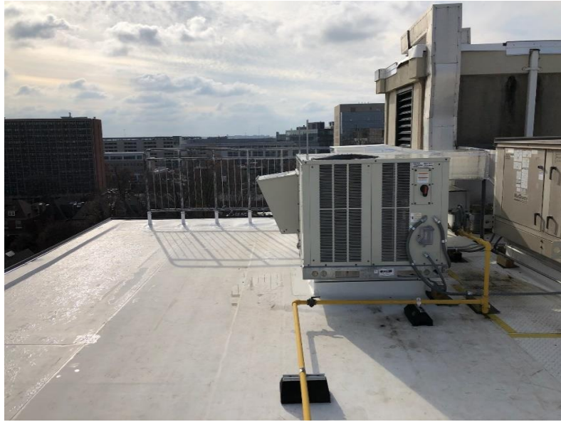
West Pine Roof Replacement
