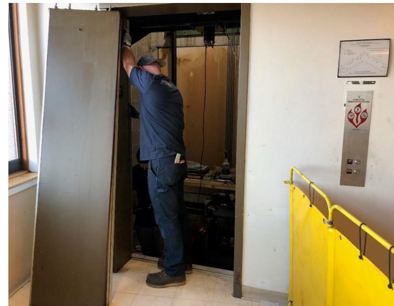
Parkview Elevator Replacment
