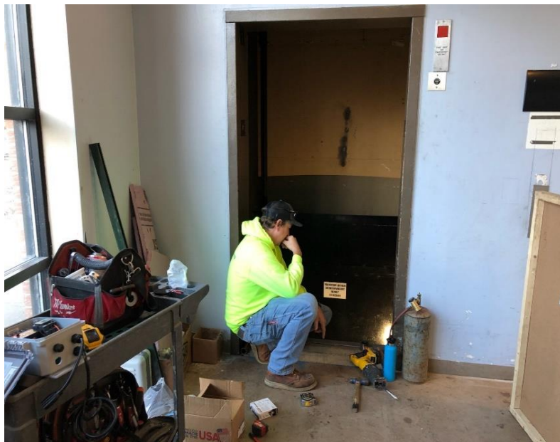
Parkview Elevator Replacment
