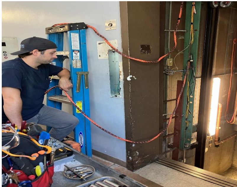
Parkview Elevator Replacement
