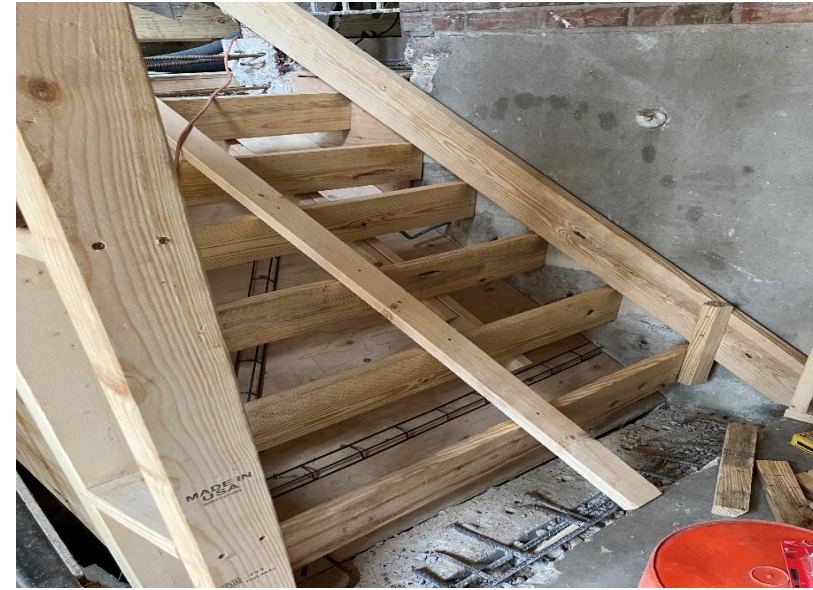
California Gardens Security Fence & Stair Repairs
