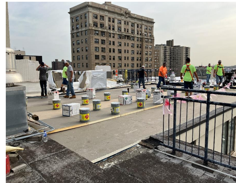
West Pine Roof Replacement
