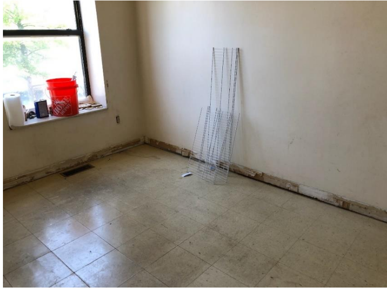
Tiffany Unit Repairs
