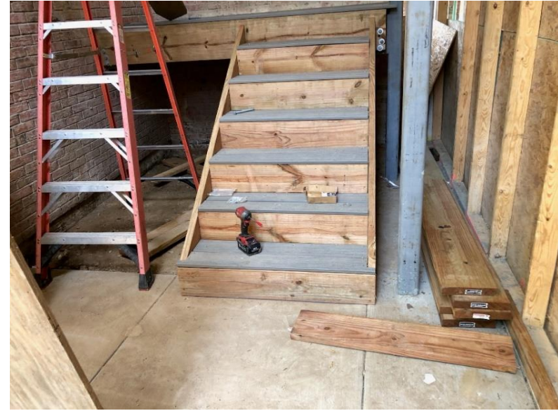
California Gardens Security Fence & Stair Repairs
