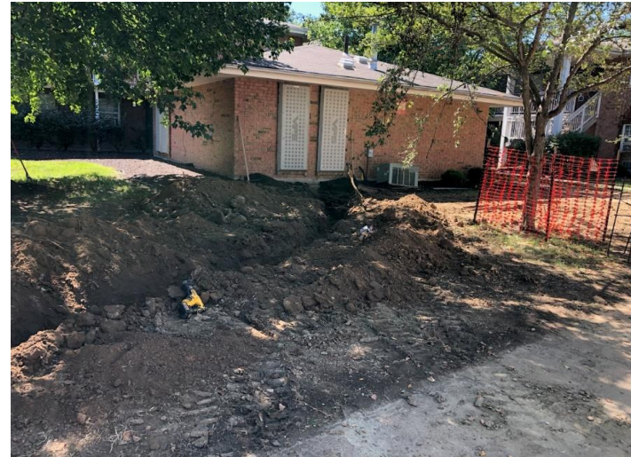
California Gardens Security Fence & Stair Repairs
