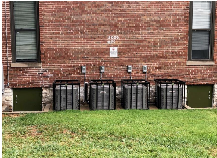
2900 Park Structural Repairs & Unit Upgrades
