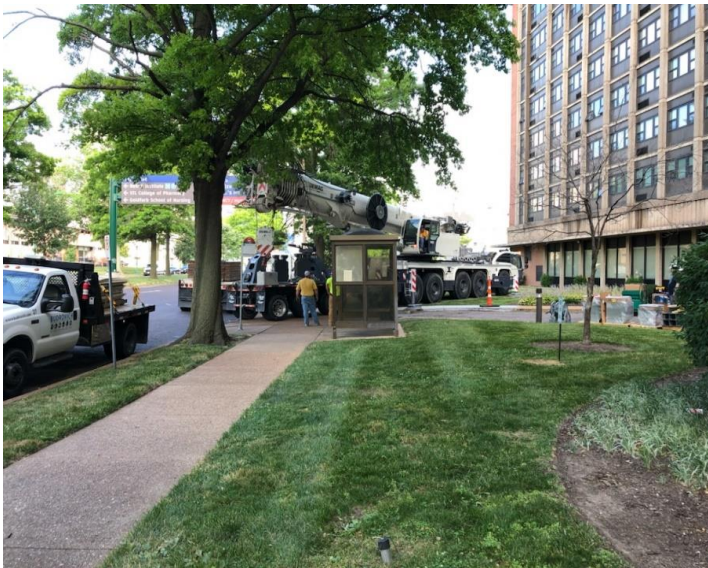
Parkview Elevator Replacment
